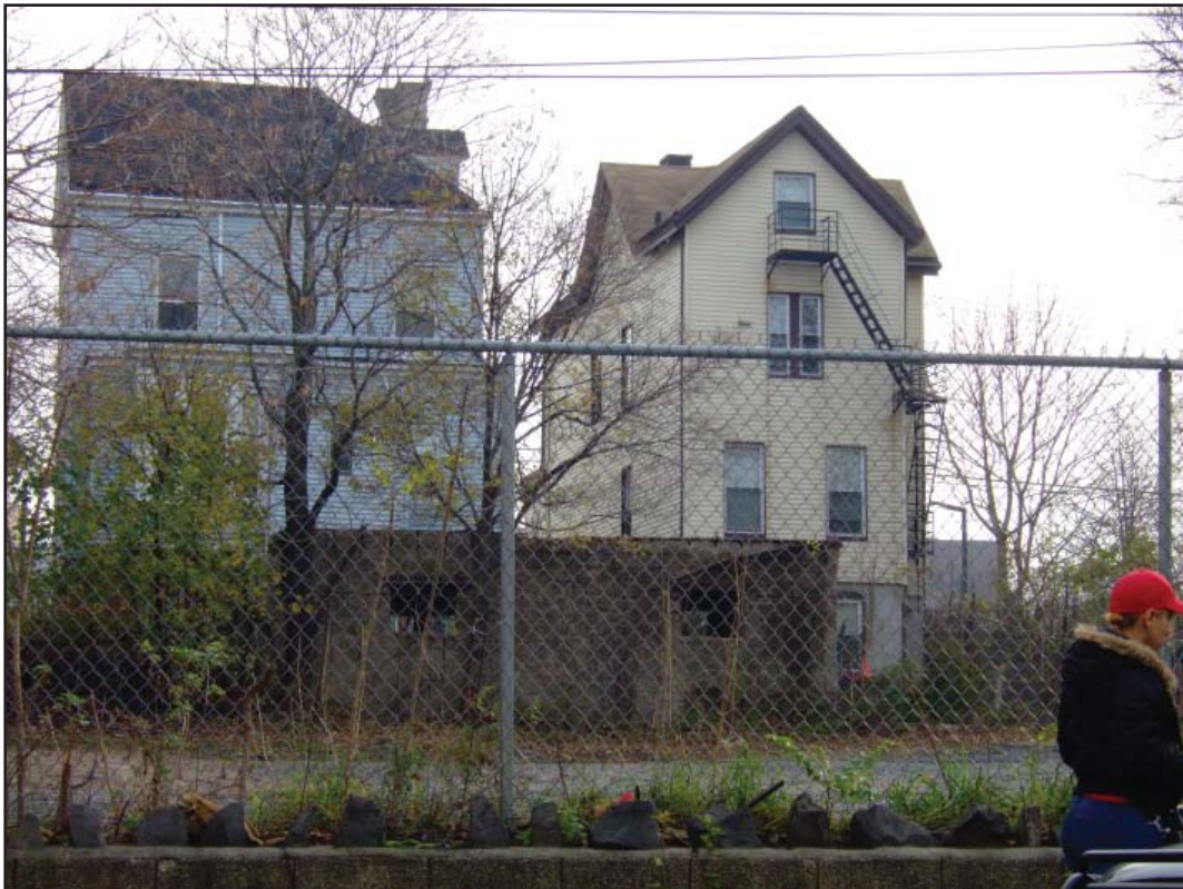
Two wood-frame residences remain on Hawthorne Avenue, with a shared garage in poor condition as evidenced by the sagging roof and unkept ground.
